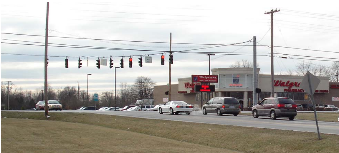
EXISTING INTERSECTION – FEGENBUSH LANE/OUTER LOOP/SOUTH WATTERSON TRACE
